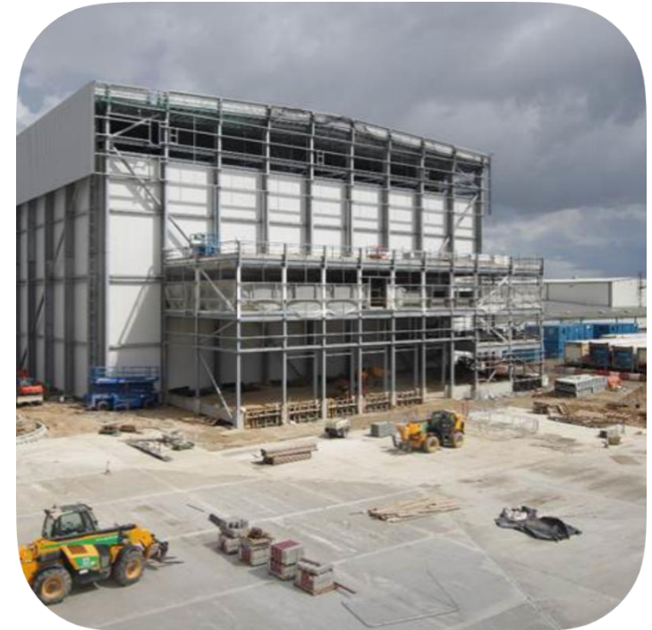
Automated frozen logistics facility on track for Q2 2021 commissioning
